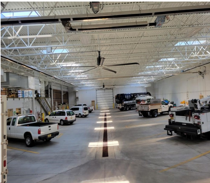
Water Utility Building
