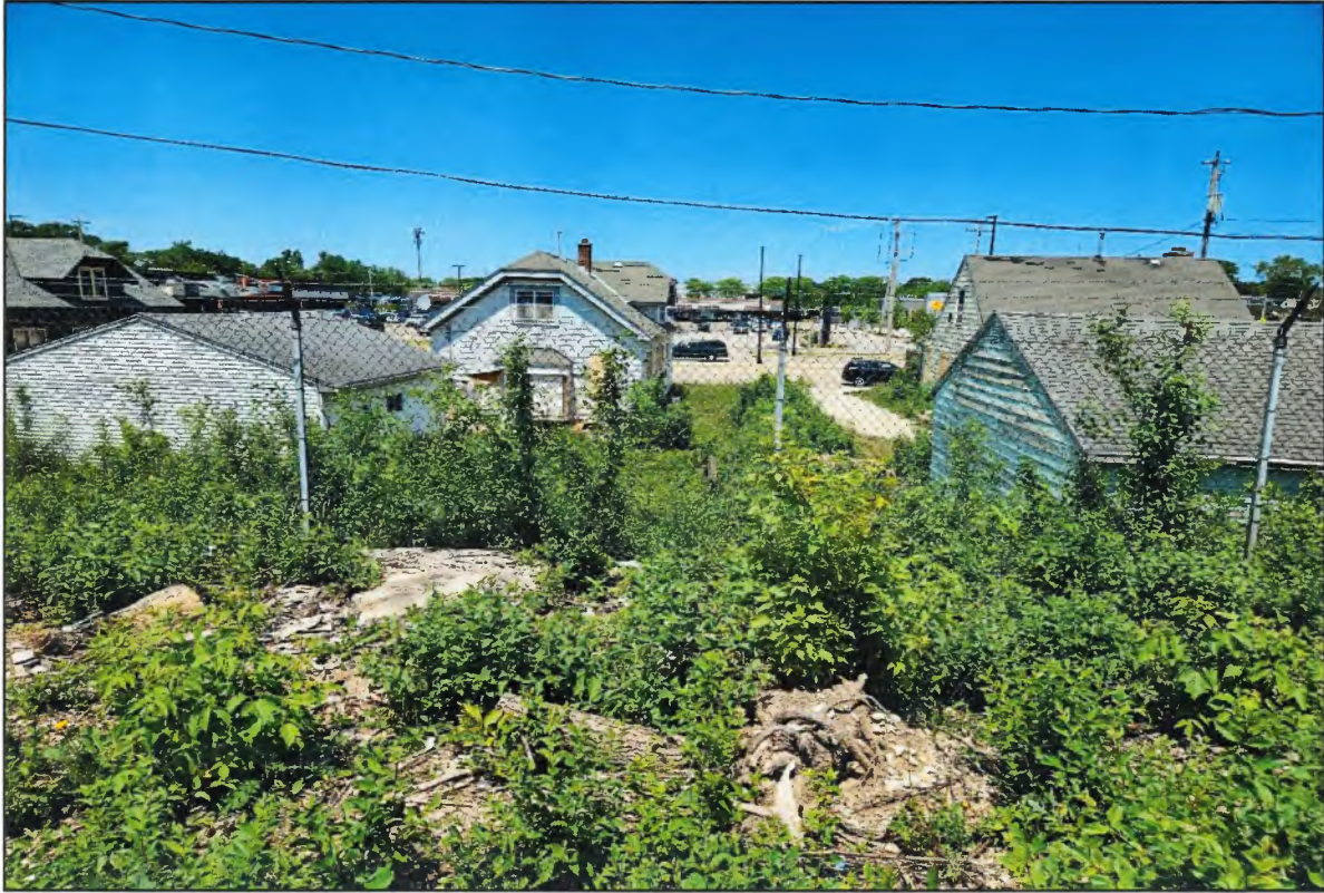
Photo 11. Rear of 2729 and 2723 W. College Ave, facing north.
