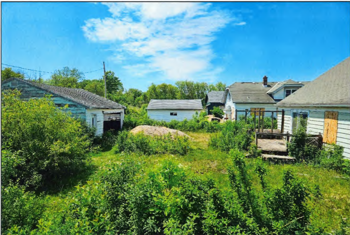
Photo 8. Backyard of 2723 (foreground) and 2729 (background) W. College Ave, facing west.
