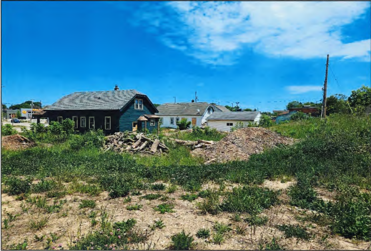
Photo 3. 2807 (foreground) and 2729 (background) W. College Ave, facing northeast.
