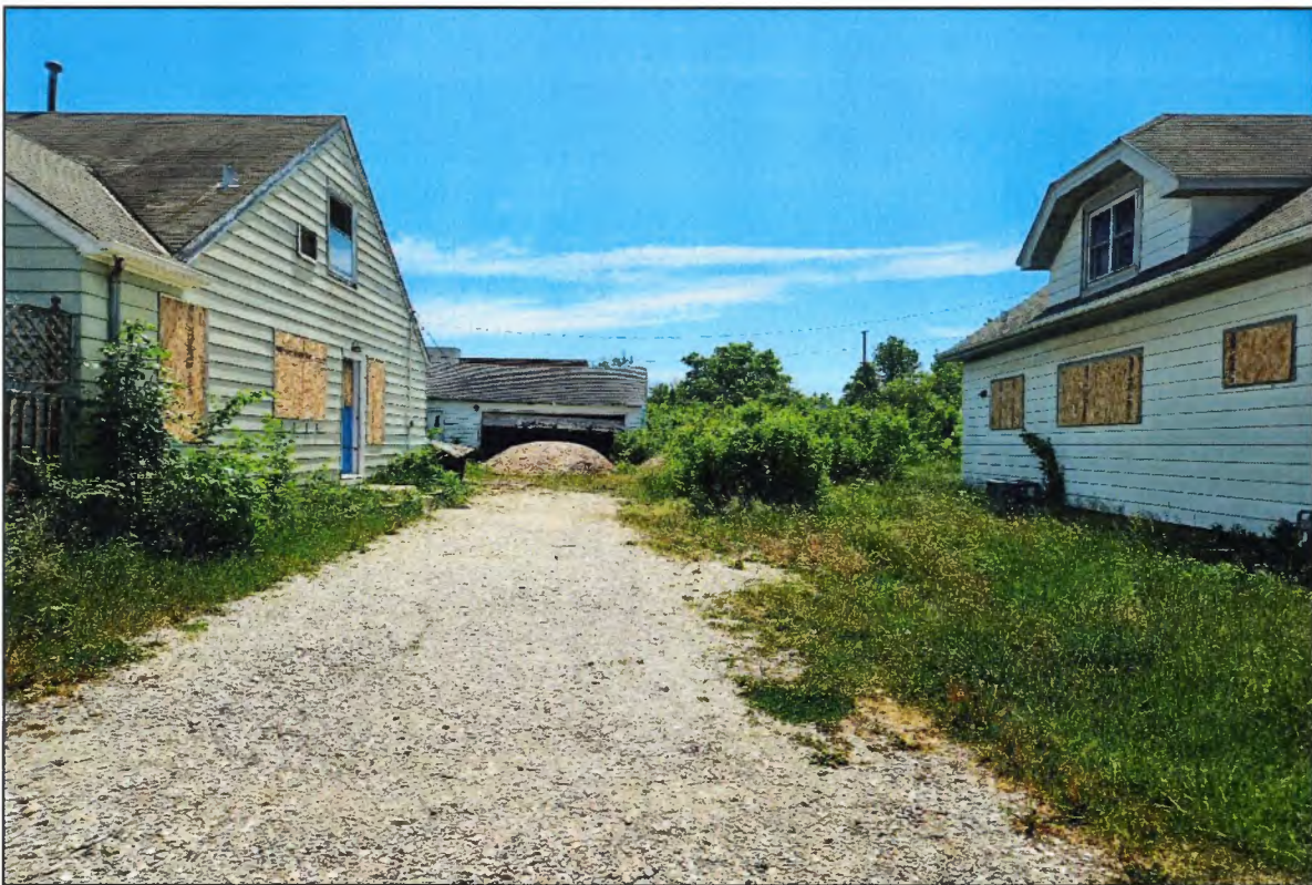
Photo 6. View between 2729 and 2723 W. College Ave, facing south.
