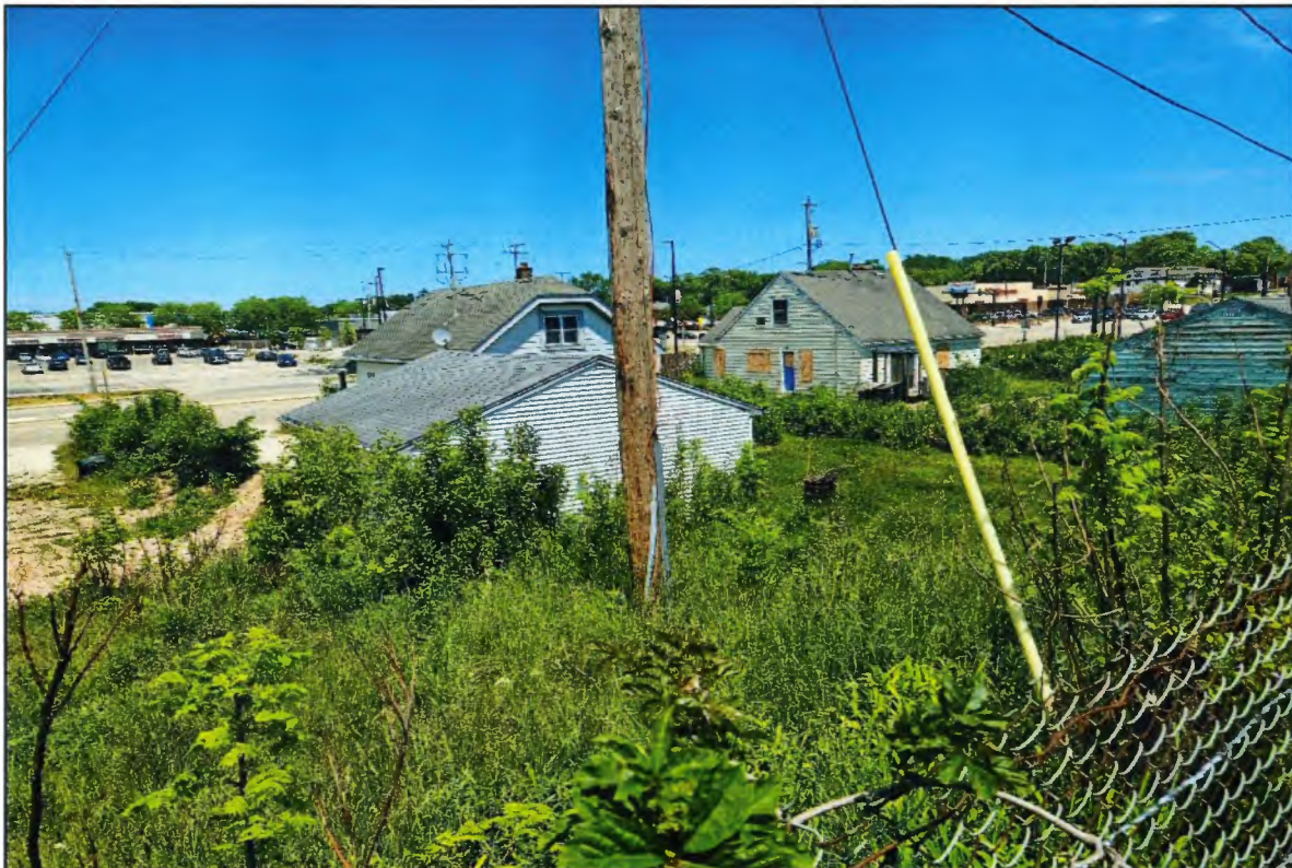
Photo 14. Rear of 2729 and 2723 W. College Ave, facing northeast.
