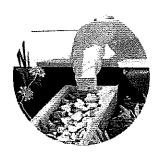
Rainwater runoff from your roof flows through the downspout into a stone-filled trough that redirects the water into removable planting compartments. The compartments contain stone and an engineered soil mix designed to filter pollutants from roof runoff and grow plants. Below the soil is a layer of stone for water storage so that plants have access to water during dry weather.
