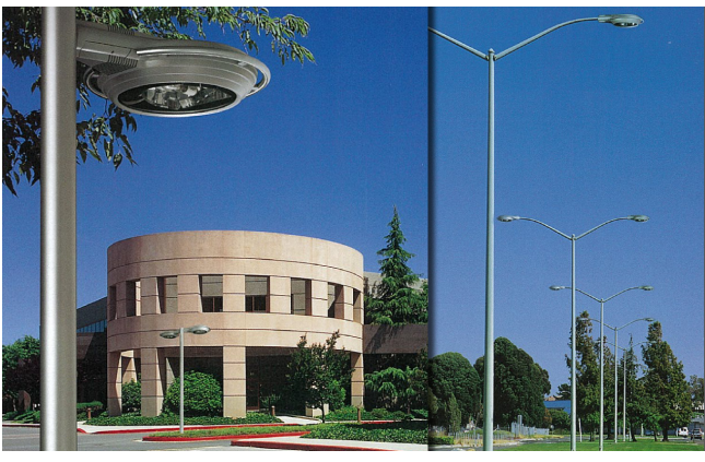
Figure 4-21: Typical roadway lighting (arm for light fixture is not needed) – Circa luminaire.
