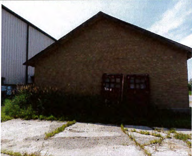
Former granary /future visitors center - east
