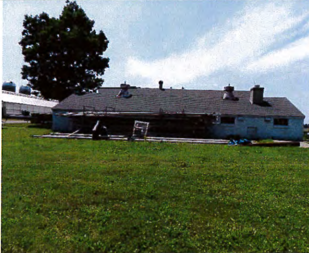
Former chicken coop /current tool shed - east
