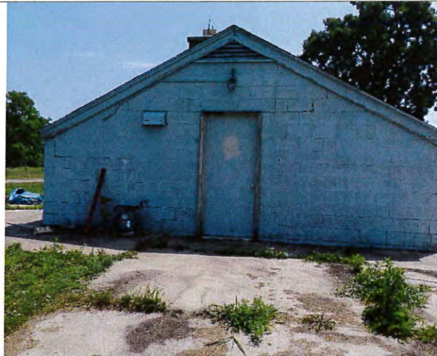
Former chicken coop /current tool shed - north
