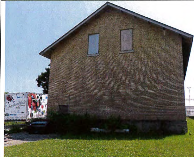
Former slaughterhouse /current tool shed - north
