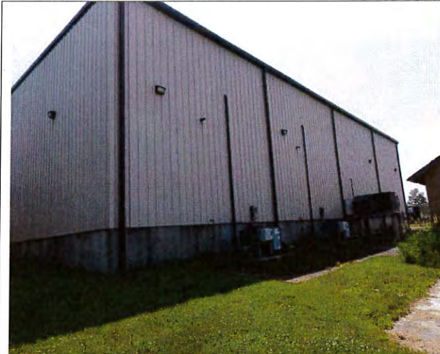
Warehouse / Harvest Haus - north
