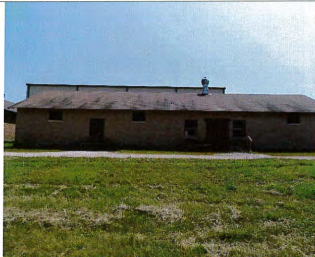
Former granary /future visitors center - north
