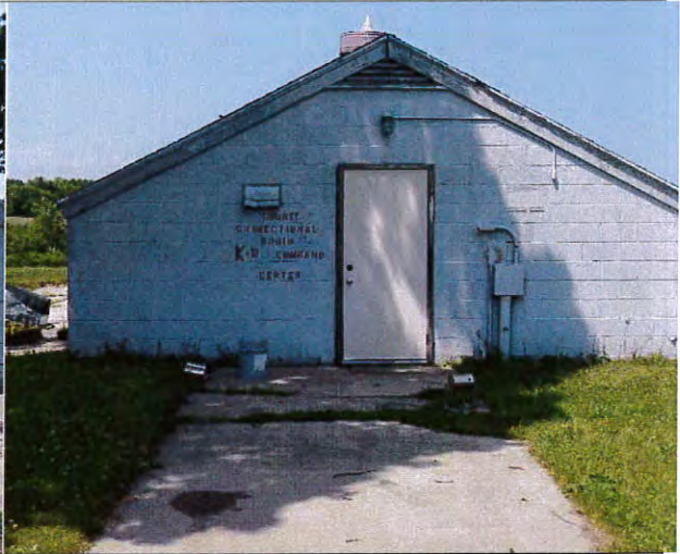
Former chicken coop /current tool shed - south
