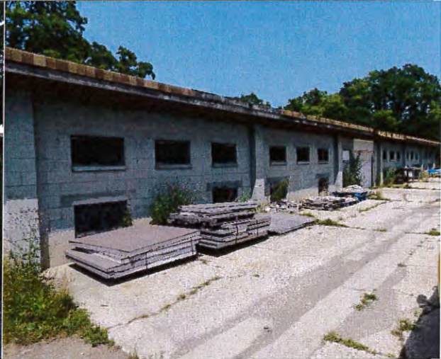
Former pig barn /current tool shed - south
