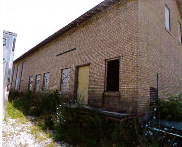
Former slaughterhouse /current tool shed - east
