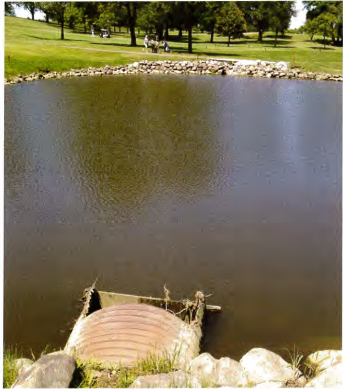
Figure 4. Dam 2, weir face on existing culvert
