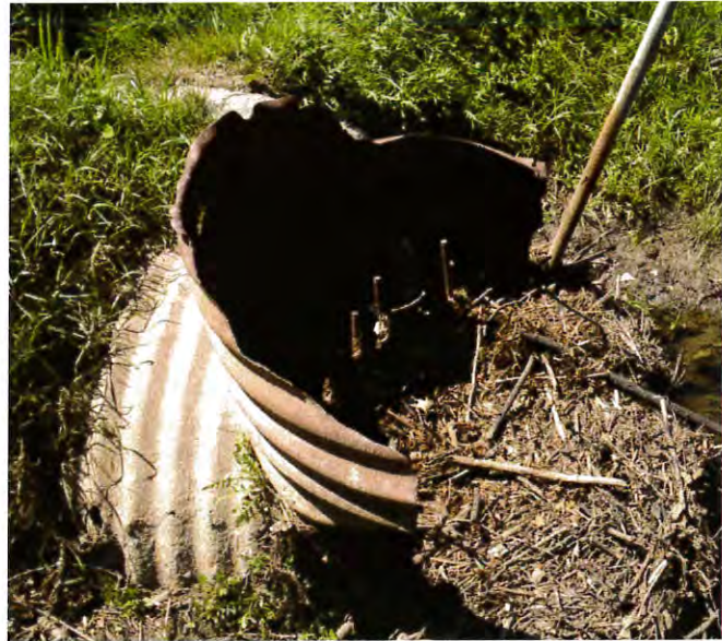
Figure 2. Dam 1, clogged and corroded
