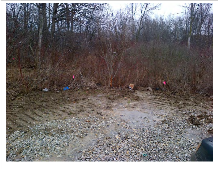
Photo 5. Southeast view of the east side of W-1 from the graveled turf area.
