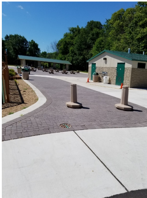
North End of Pavers (looking south)
