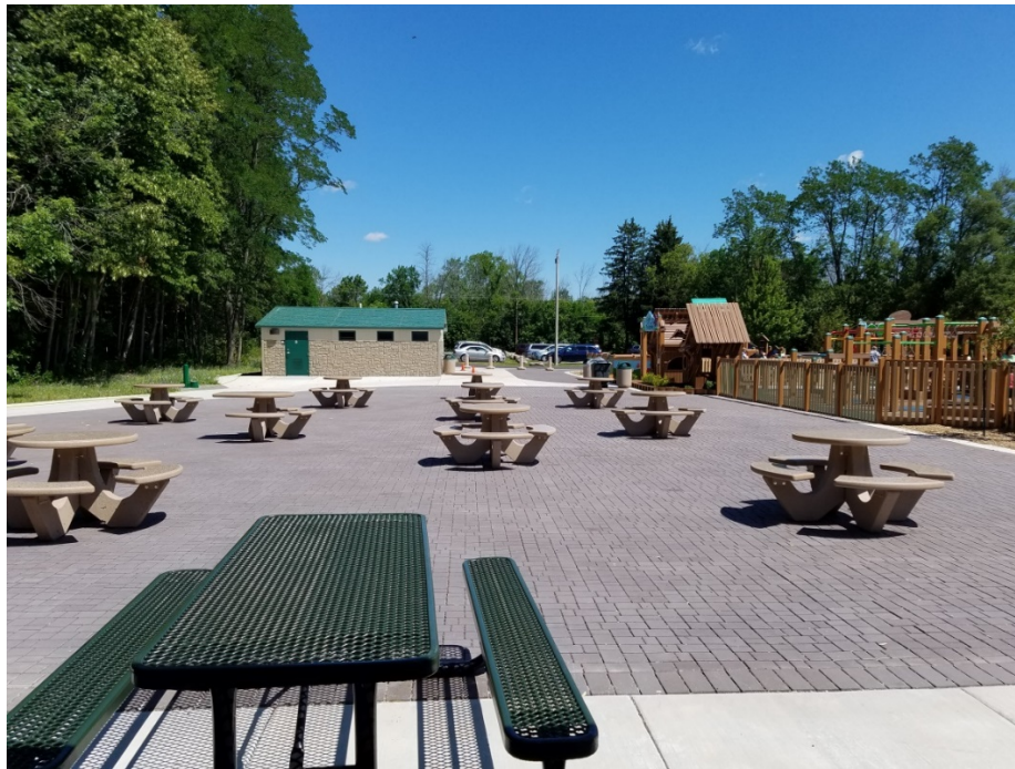
South End of Pavers (looking north)
